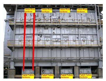
Photo showing location of multiple reformer tube rows and pigtail tube sections within a single firebox reformer.
