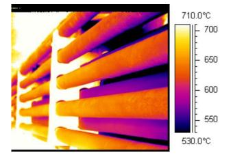
There are also the "pigtail" tubes of a reformer which can be inspected. Pigtail tubes are the smaller tubes that are external to the furnace and connect the reformer tube to the supply and exit manifolds.
