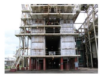
Foster Wheeler horseshoe type design: One row of tubes per firebox/cell
