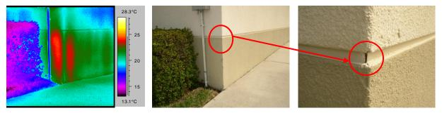
Figure 18. Image on left shows trapped moisture in a stucco wall system below a control joint. The right image shows an opening in the joint at a corner seam that is allowing water to enter the wall
