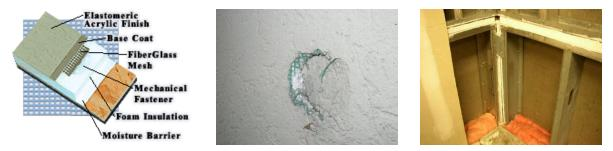
Figure 10. Cutaway diagram at left showing main components in an EIFS construction (image courtesy of Total Wall Inc.). Middle photo shows the exterior finish, fiberglass mesh and internal foam. Photo at left shows exterior drywall fastened to metal stud wall system.
