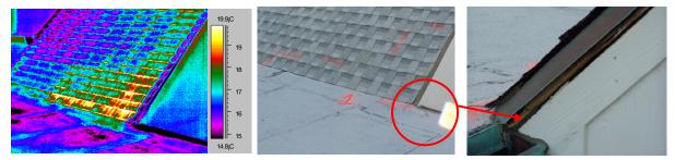
Figure 22. Infrared image showing trapped moisture (orange areas in images) beneath a shingle roof system. Edge metal flashing was not installed correctly and allowed for moisture to enter the wood deck
