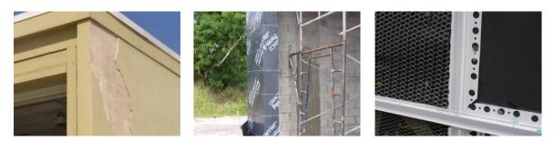
Figure 15. Image on left shows direct applied stucco over CMU that is de-bonding. Middle image shows vapor barrier directly applied to CMU prior to metal lath and stucco finish. Image on right shows mechanically fastened metal lath and control joint bands applied over moisture barrier and CMU
