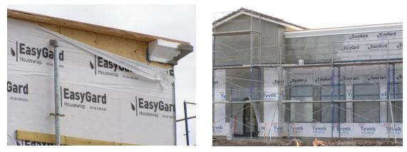
Figure 19. Image on left shows wood framed commercial building with vapor barrier applied. Note the foam trim piece applied in the upper right corner to make up the eave of the building. Image on right shows stucco being applied over metal lathing on a different section of the building
