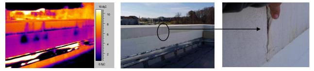
Figure 12. Infrared image shows migrating and trapped moisture. Middle image is control picture showing location of one of several areas where caulk joint is open as shown in right image
