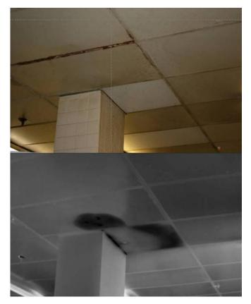
Figure 9. Uninsulated structural components, such as a column, may pass from a cool area into the interstitial space causing condensation on the column which drips onto the ceiling
