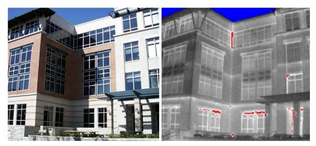
Figure 4. Visual and infrared images of an office building showing air leakage
