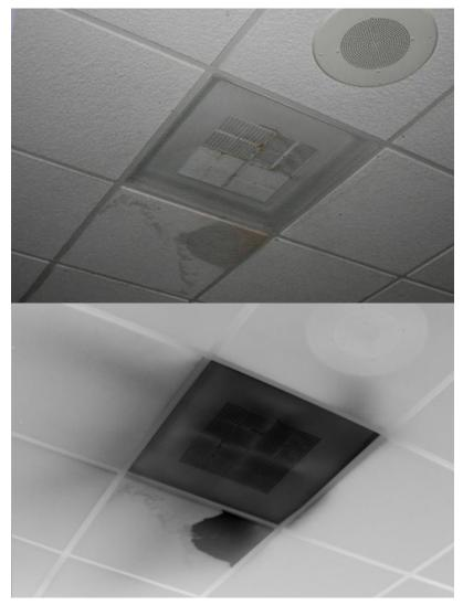
Figure 7. Often, ductwork is not sealed well or not fastened tightly to the diffusers, which allows cool air to blow into the warmer interstitial space, creating condensation that drips onto the acoustical ceiling tiles
