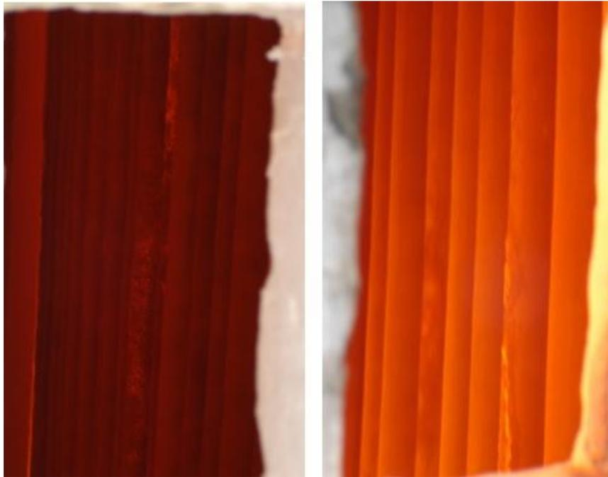
**Figure 5: Visible Color Change of Tubes Due to Temperature**
