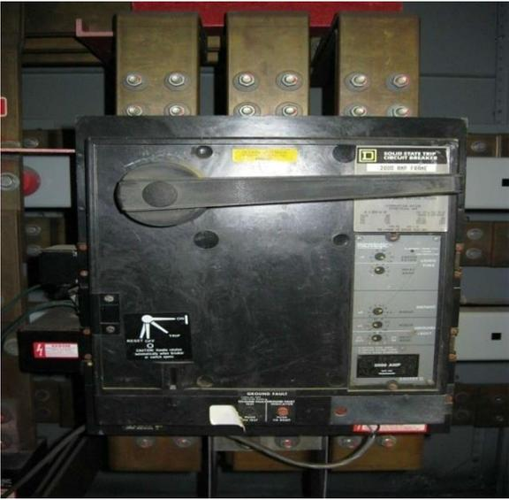
The image above is a 2000 amp main breaker. Arcing was detected on the B-phase line side. The arcing heard was worse when the load increased. The arcing has severely deteriorated the internal contacts, and eventually will become so deteriorated that the voltage and wave form will be unable to reach the load. At this particular facility, the replacement cost for this item is approximately \$20,000 USD.
