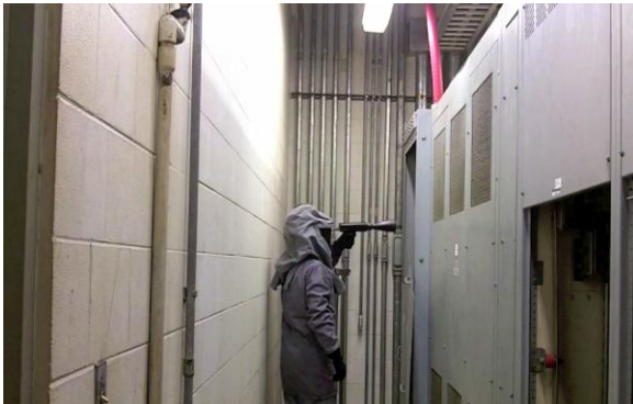
Ultrasound inspection in progress
