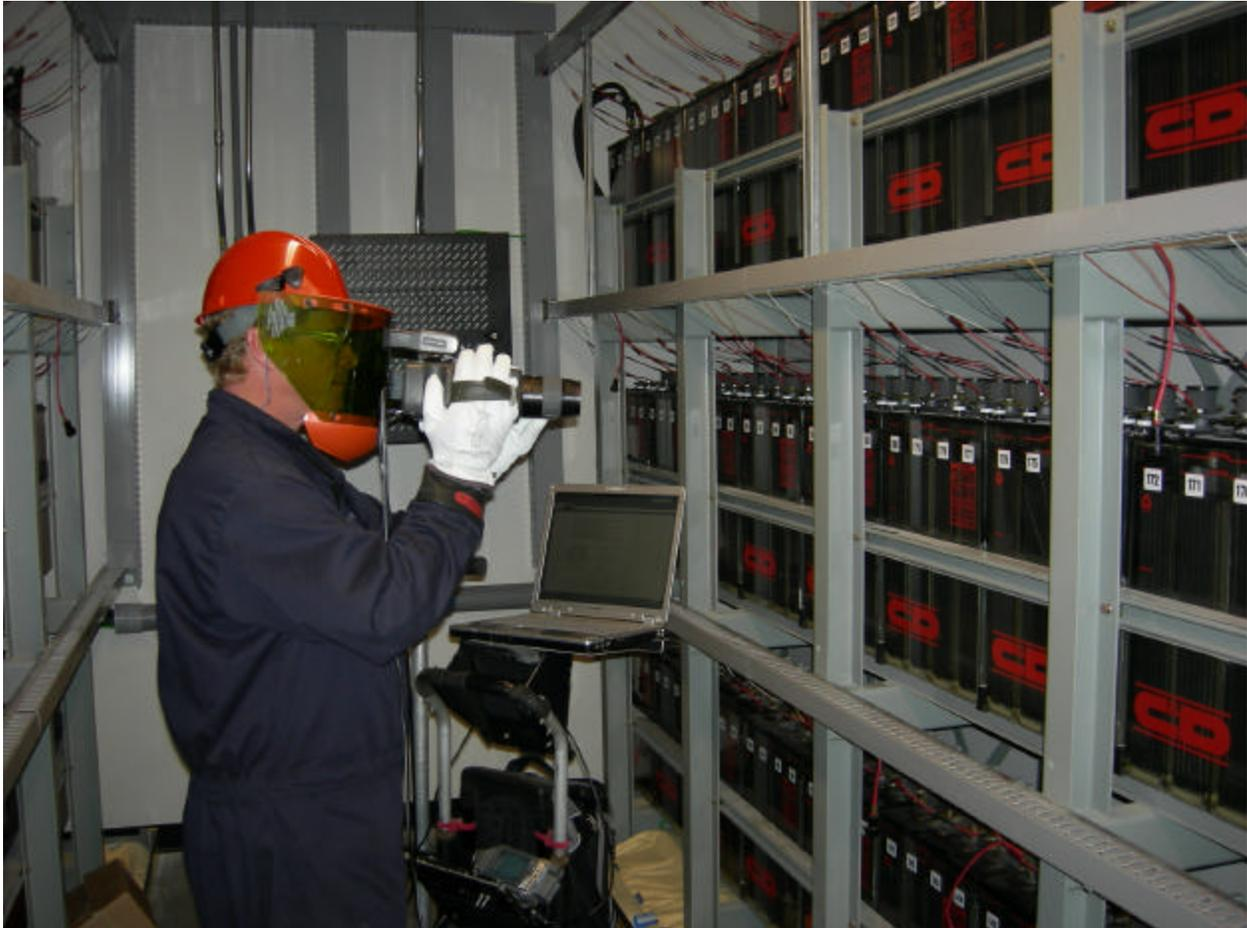
Figure 5. Thermographer inspecting a battery bank during full battery discharge testing
