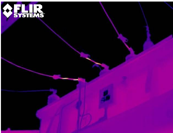
Figure 3. High resolution thermal image of a 115kV to 23kV substation transformer low side. Significant thermal anomaly on left and center phase jumpers due to some strands broken or poorly connected. IR image effect is often termed “barber poling”.
