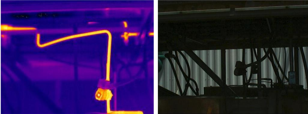
**Compressor Oil Line Solenoid Valve**
