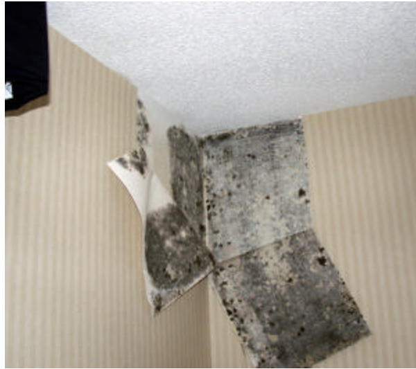
Figure 2c) Visual image with mold present
