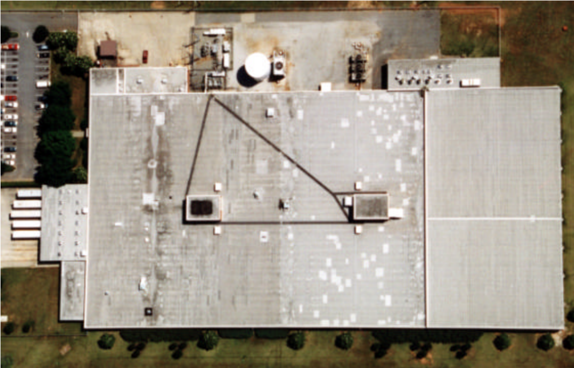
Figure 8) Visual photograph of a roof.
