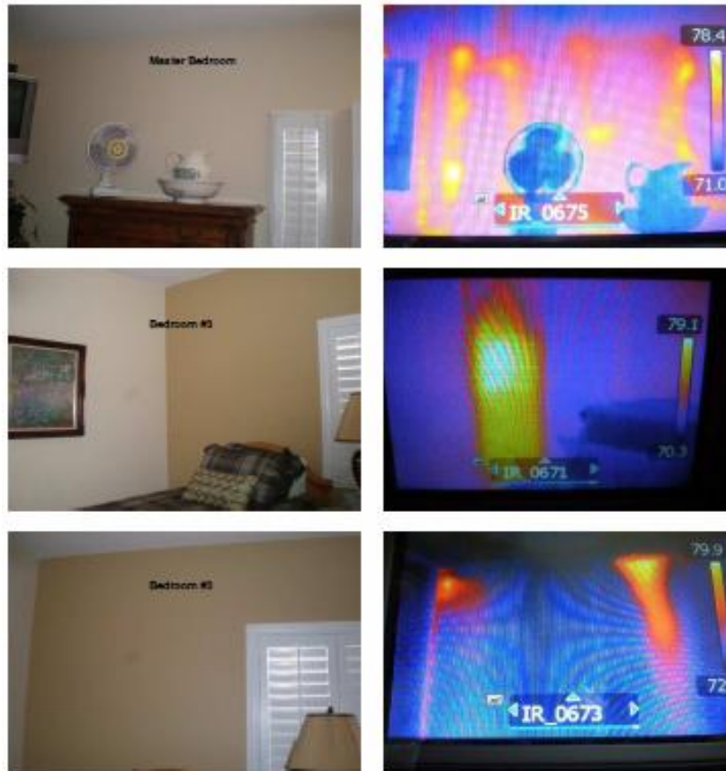
Example of a poorly conducted survey and an inadequate report taken from an unnamed report. These images represent the entire thermographic section of a report taken during a home inspection.
