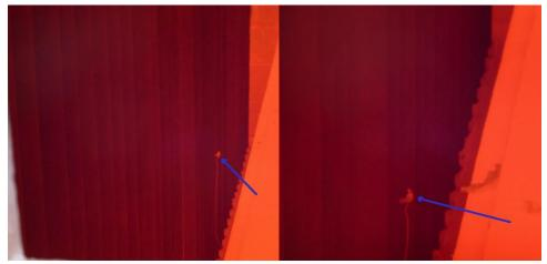
Figure 6: Embedded Thermocouples on Reformer Tubes
