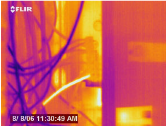
Above thermal and daylight images show an overheated neutral on the neutral bus bar of a distribution panel, most likely due to harmonics.
