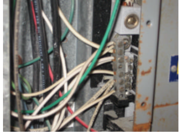
Above thermal and daylight images show an overheated neutral on the neutral bus bar of a distribution panel, most likely due to harmonics.
