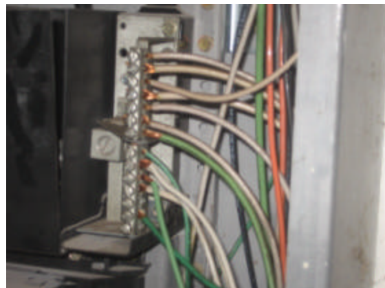
Above thermal and daylight images show overheated neutral wires, proven to be caused by harmonics.
