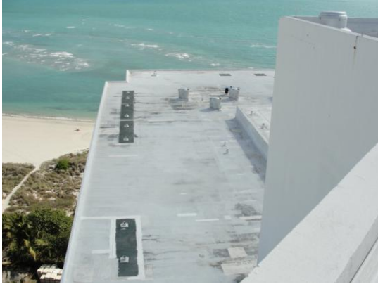
Figure 1: Ocean front condo with very low parapet wall on a flat roof system. Roofs like this can cool very quickly shortly after sunset, if there is wind coming off the water.
