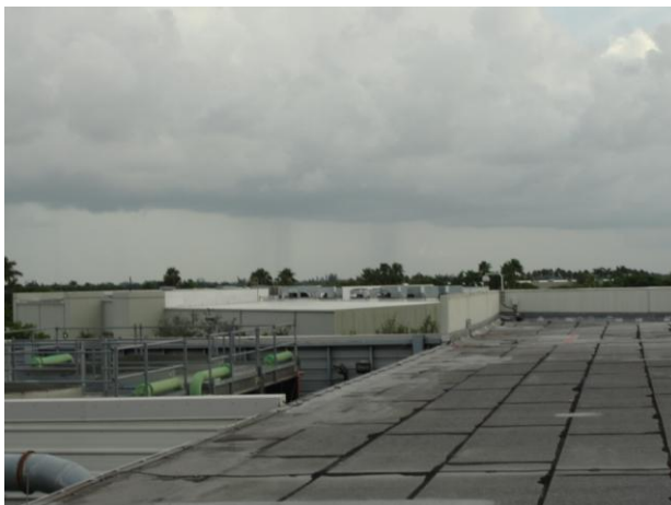
Figure 2: Overcast skies with rain showers around job site created an early and short-lived scanning window on this roof. Scanning took place between 3:30 PM and 5:30 PM.
