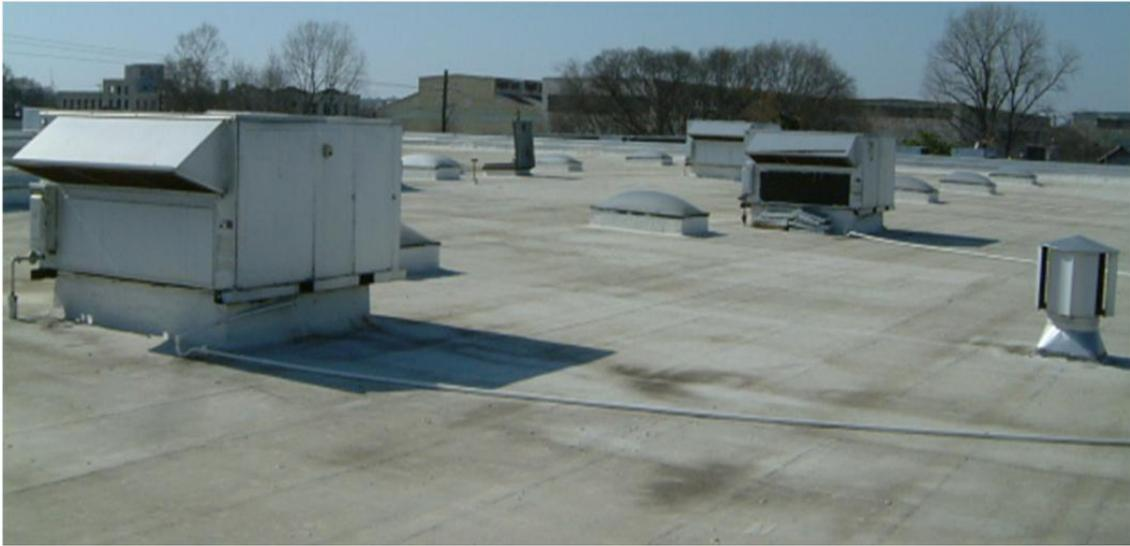
**Figure 1) – Typical low-sloped insulated roof**
