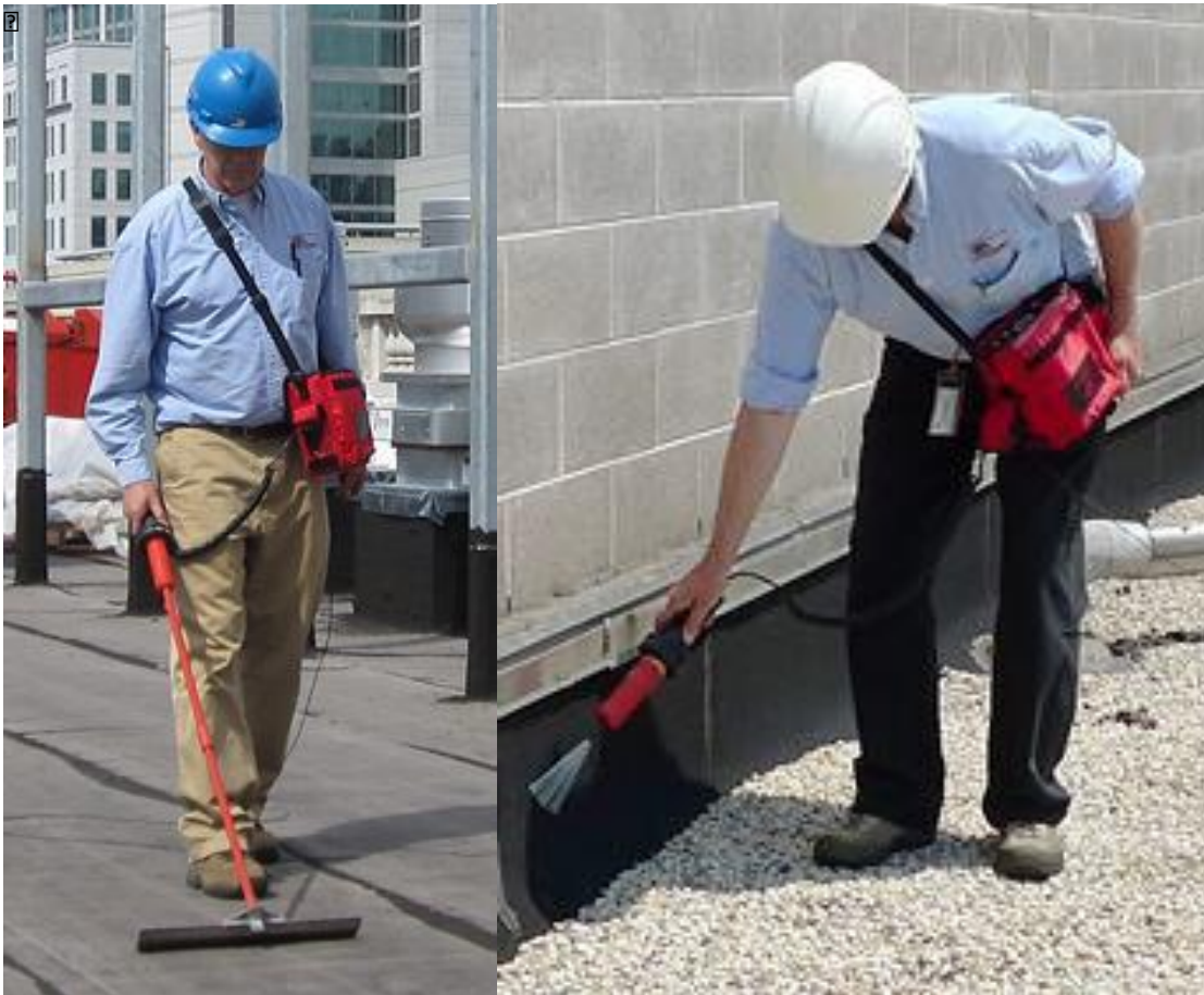
Figure 4: High voltage testing on both horizontal and vertical membranes. (Images Courtesy of IR Analyzers)
