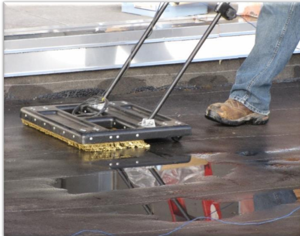
Figure 5: Low voltage scanning platform being pushed across horizontal membrane.
