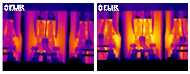
Figure 6. Medium resolution (left) and low resolution IR images of 480 volt generator tie-in breaker.
