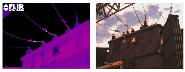
Figure 3. High resolution thermal image of a 115kV to 23kV substation transformer low side. Significant thermal anomaly on left and center phase jumpers due to some strands broken or poorly connected. IR image effect is often termed "barber poling".
