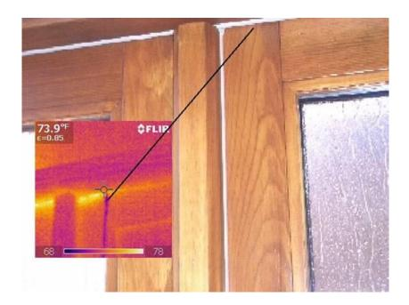
This is easy to discover and the repair / remediation process is standardized by the factory. The thermogram that follows shows a glazing juncture failure where water is coming around the bottom of the insulated glass unit (IG) on a door.
