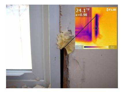
The unit above was found to have a void in the insulation at the bottom of the rough opening. The initial scan showed a cold anomaly and removal of the casing proved this.
