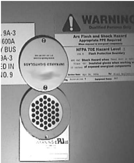
Fig 4. Universal IR port and warning labeling
