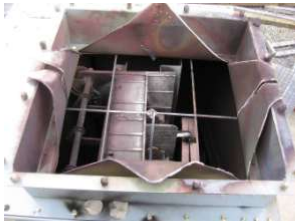
Fig 14. Pressure relief plate after an arc-flash event
