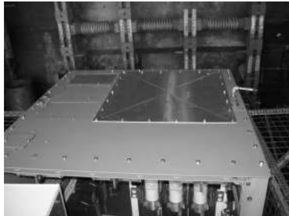
Fig 11. Pressure relief plate
