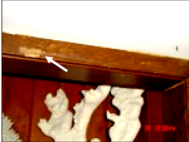
The left photo is the site of drywood infestation and the right photo is replaced wood, which was once infested. As you can see, the wood color does not quite match up.
