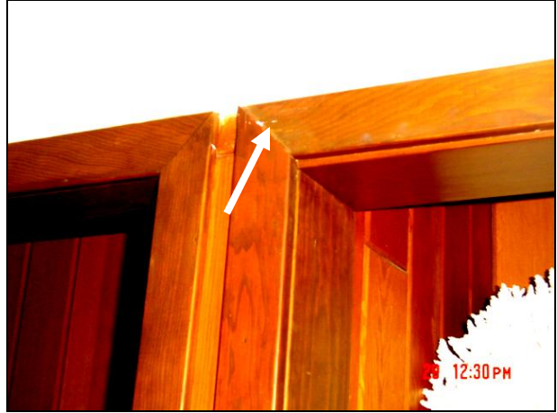
The left photo is the site of drywood infestation and the right photo is replaced wood, which was once infested. As you can see, the wood color does not quite match up.
