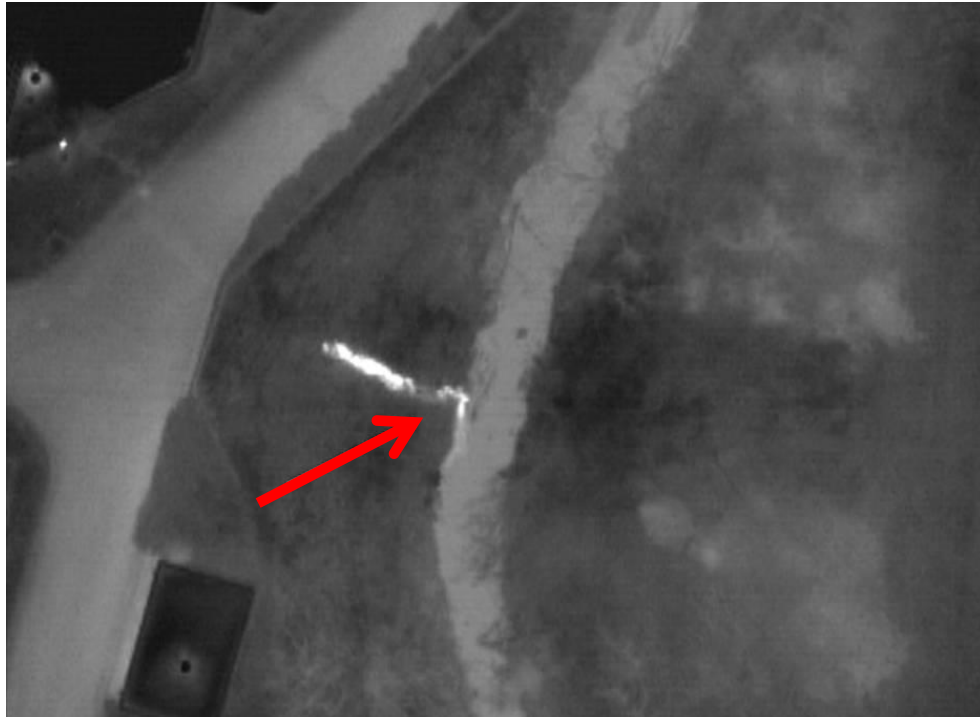
Figure 7. IR image of a storm water drainage system outfall flowing into a creek
