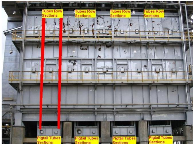
**Photo showing location of multiple reformer tube rows and pigtail tube sections within a single firebox reformer.**
