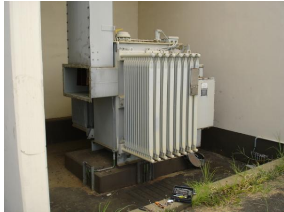
Low oil level results in no oil circulating through transformer's radiator fins and windings overheating
