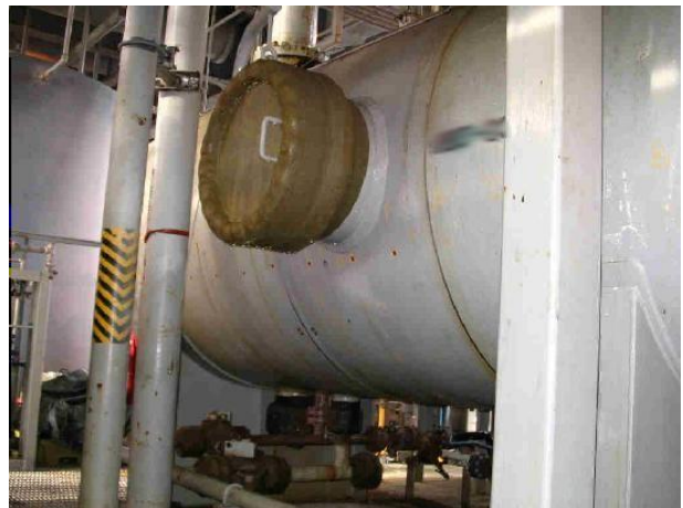
Separator's outlet section showing solids (sand) exiting the outlet piping
