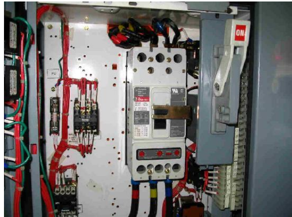
480V MCC breaker with damaged cable
