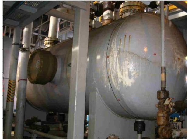
Separator's inlet section showing solid (sand) and fluid (water, oil, & gas) levels
