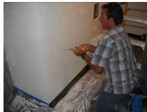
Opening of wall to prepare for testing
