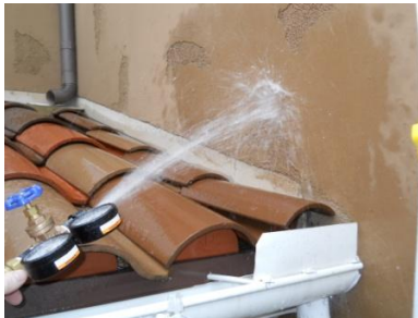
Water testing suspected area
