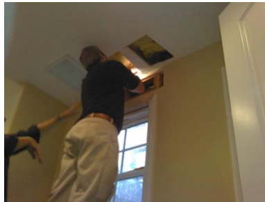
Cutting openings in ceiling
