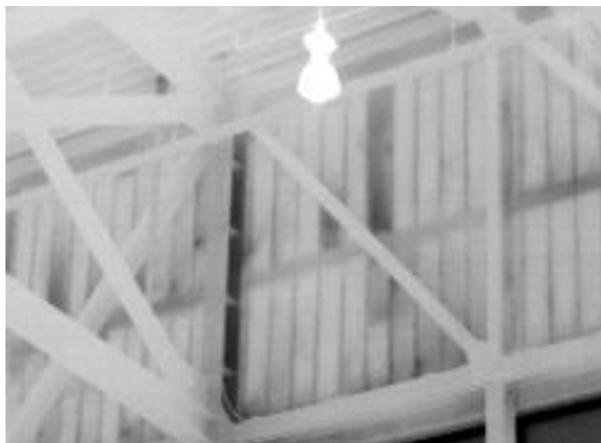
**Figure 2. Infrared image of a convention center wall with missing and misplaced fiberglass batt insulation (darker areas)**
