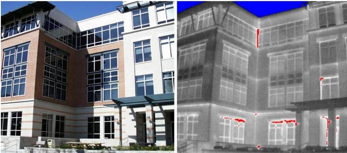
**Figure 4. Visual and infrared images of an office building showing air leakage**
