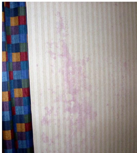
**Figure 11. Visual image of the inside of a hotel exterior wall with non-perforated vinyl wallpaper showing stains from mold**
