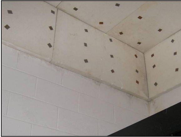
Figure 10. Insulation pinned to a below grade CMU wall
