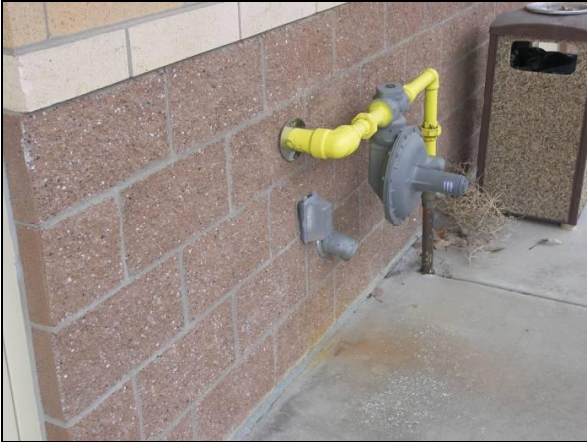
Figure 26. Electrical and gas utility penetrations in the enclosure
