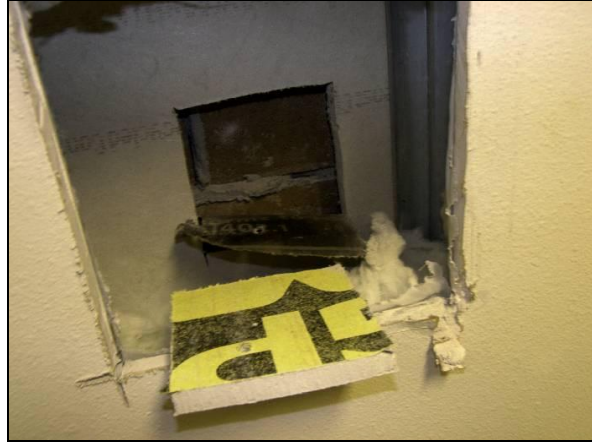
Figure 31. Invasive investigation reveals actual as-built conditions. Additionally, as each material is carefully excavated, a pressure differential can be measured between material planes which helps to understand the root cause of failure in a forensic investigation of an air barrier system
