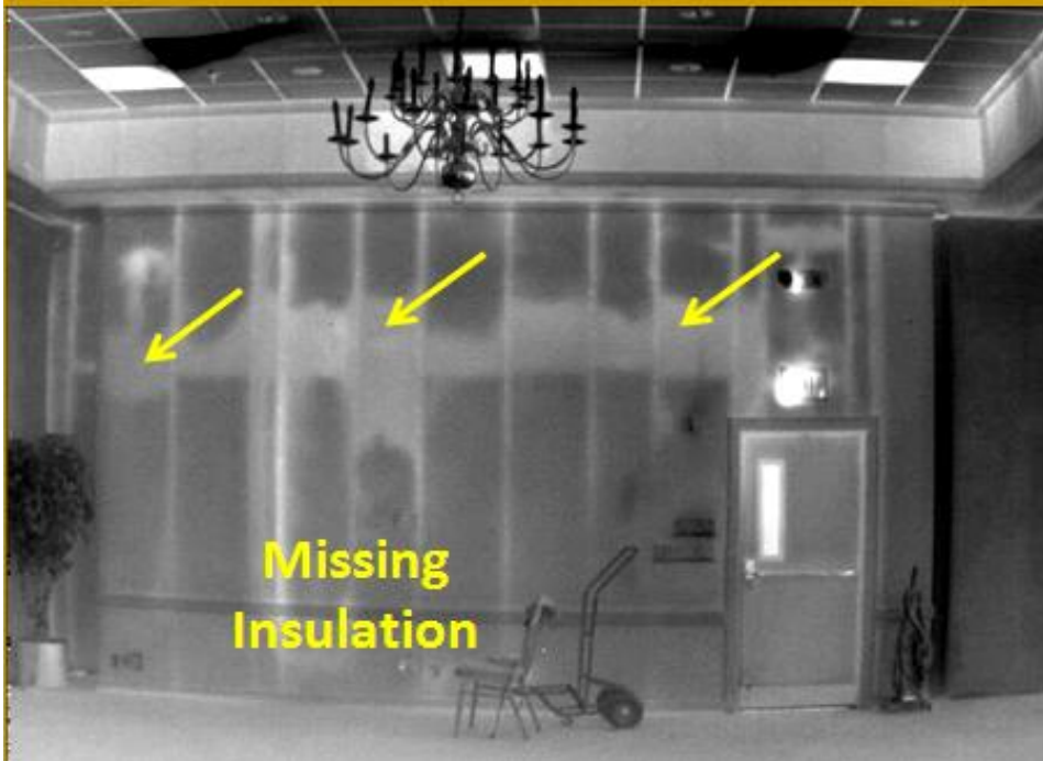
Large Building Insulation Surveys – Hotels/Libraries
