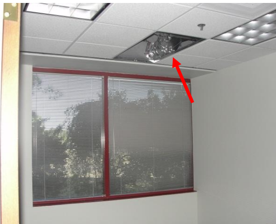
Figure 10 (right): Typical office space showing two ceiling tiles removed to promote proper air flow throughout building.
