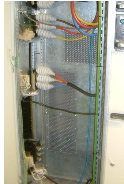
Figure 6: IR transmissive screens
