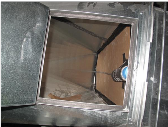
Figure 34. Temporary air sealing inside stairwell air supply ductwork
