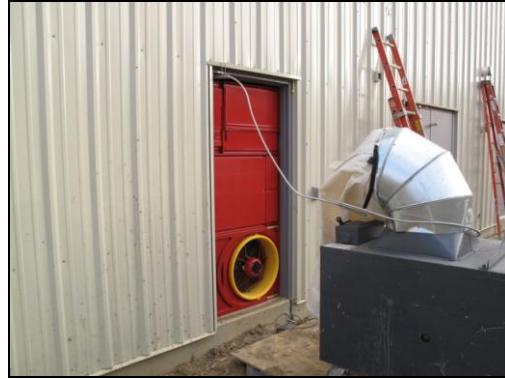
Figure 5. Single fan units can be used to pressure test small buildings
