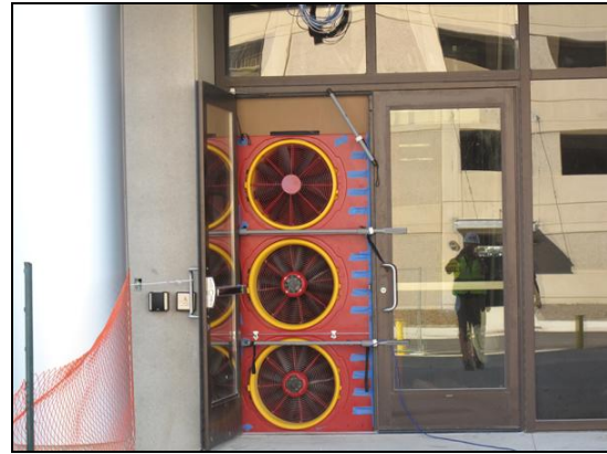
Figure 33. Door fans set up in the North exterior door
