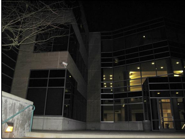
Figure 24. Exterior storefront and brick panel system of an office building
