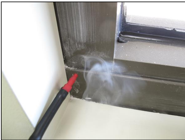
Figure 30. A smoke puffer is used to verify air leakage at a window assembly
