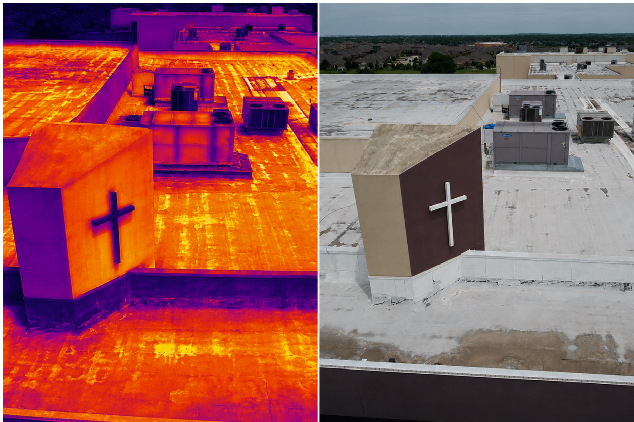
Figure 3. The same roof viewed in thermal infrared (left) and visible light (right). The thermal image records surface temperature patterns, while the visible image reveals construction details, coatings, drainage, and equipment. Neither image explains the observed anomaly by itself. Defensible conclusions emerge only when thermal measurements are interpreted within the context provided by the visible inspection and field observations.
