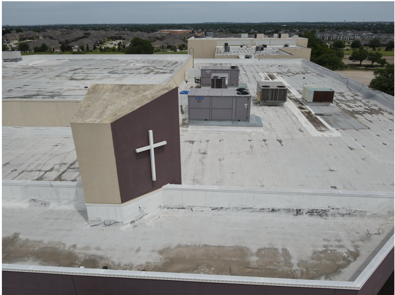
Figure 4. Cross/parapet church (visible, oblique). The headwall, elevation change, HVAC equipment, and drainage patterns are all readable from the air before landing. This is the reconnaissance walk from altitude - context building before measurement begins.
