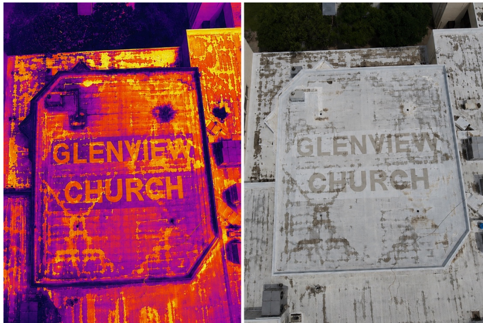
Figure 1. A thermal image records temperature patterns. The visible image reveals roof construction, coatings, repairs, drainage, and surface condition. Neither image explains the anomaly by itself. Context transforms measurements into evidence.
