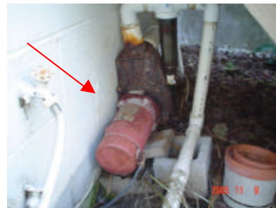
Replace pump and motor
