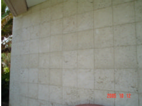
Chambers east exterior wall
