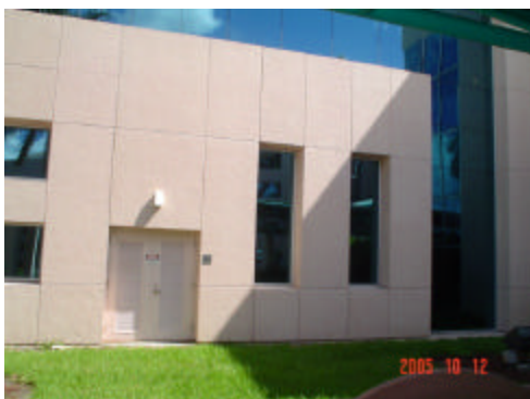
City hall south wall power room
