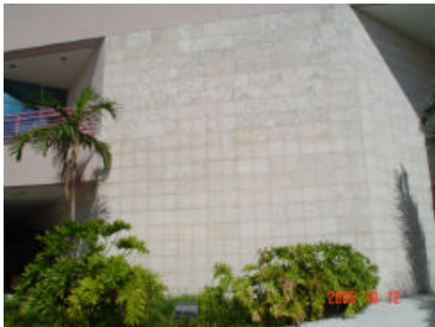
Chambers south exterior wall
