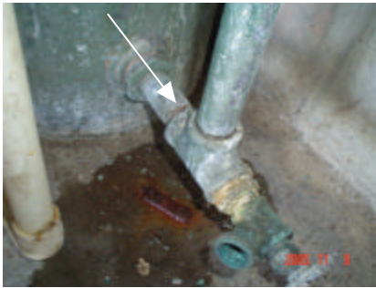
Leaking pipes
