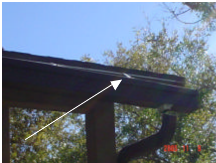
Gutter damage
