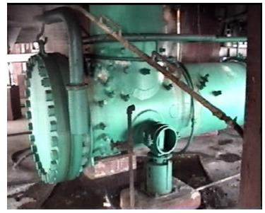
Visible Example of Steam Cooling & Injectable Refractory Nipples
