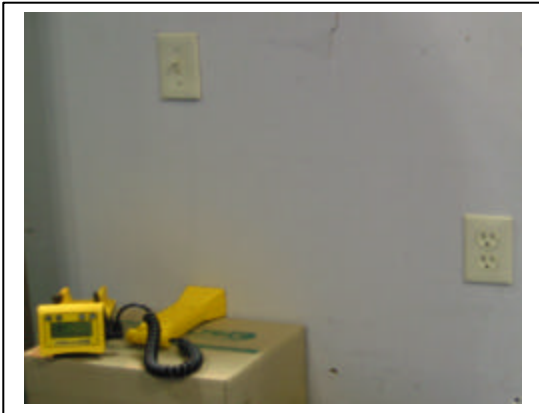
Wall face showing Termatrac in use
