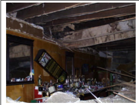
Above are two views of the Le Dale Hotel and Bar ceiling that collapsed from Formosan termite damage. Courtesy Jack Leonard – New Orleans
