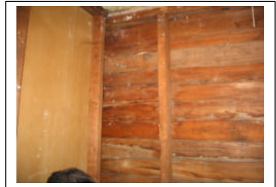
Digital image of exposed interior stud
