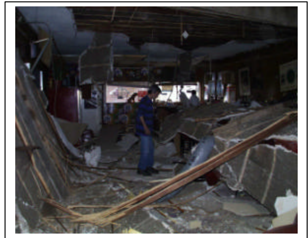
Above are two views of the Le Dale Hotel and Bar ceiling that collapsed from Formosan termite damage. Courtesy Jack Leonard – New Orleans.
