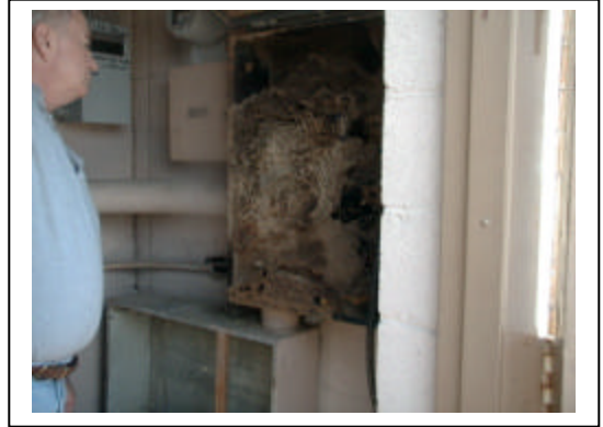
Insect pests have been known to infiltrate electrical panels. The termite carton nests above can pose serious problems. Jack Leonard – New Orleans.
