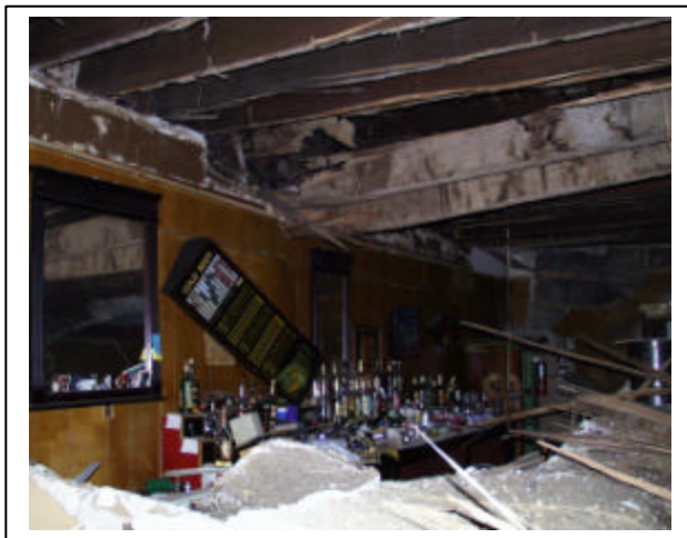
Above are two views of the Le Dale Hotel and Bar ceiling that collapsed from Formosan termite damage. Courtesy Jack Leonard – New Orleans.
