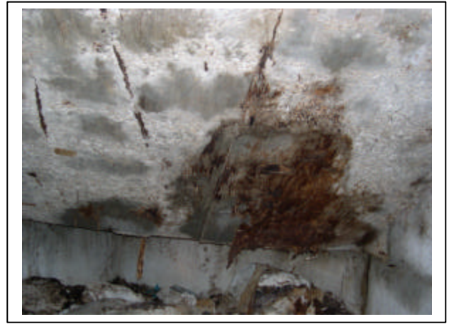
Active mold in crawl space located in Miami, FL.
