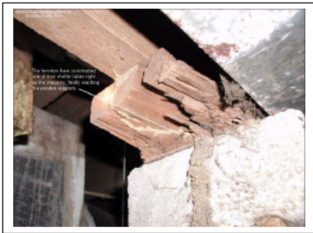
Crawl space area visually showing presence of termite mud tubes both of active and inactive nature. Courtesy – Advance Tech Pest Management, Clermont, FL.
