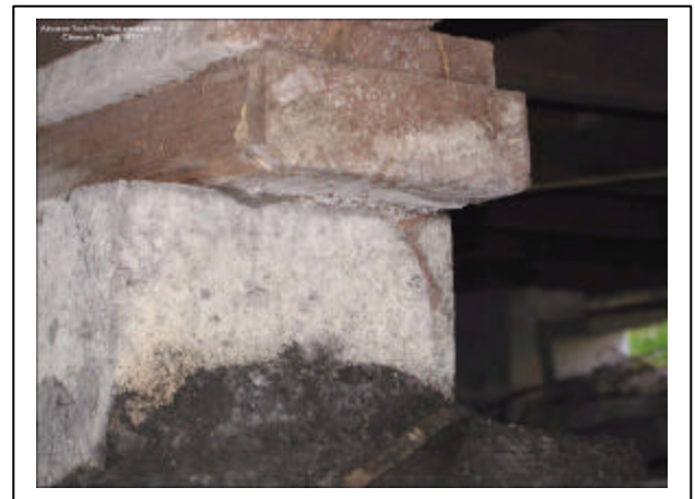
Crawl space area visually showing presence of termite mud tubes both of active and inactive nature. Courtesy – Advance Tech Pest Management, Clermont, FL.
