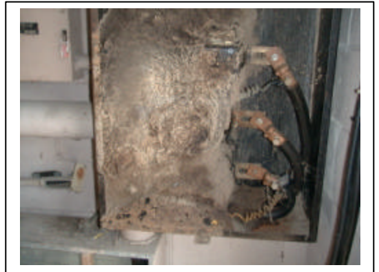
Insect pests have been known to infiltrate electrical panels. The termite carton nests above can pose serious problems. Jack Leonard – New Orleans.
