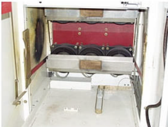
Front side of cabinet with carbon residue and electrical flash-over on breaker
