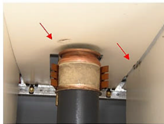
Carbon tracks on insulation between B- & C-phase fuses
