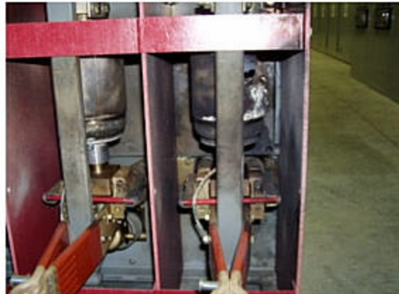
Front side of cabinet with carbon residue and electrical flash-over on breaker
