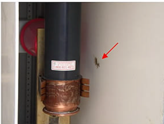
Carbon tracks on insulation between B- & C-phase fuses
