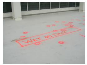
Wet/damaged roof from airborne roof tiles
