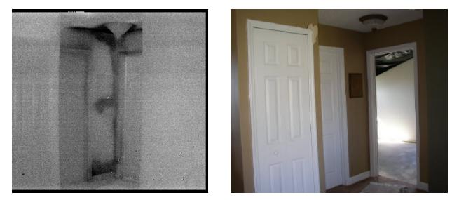
A cold thermal pattern on wall and ceiling of a residential home that suffered water intrusion
