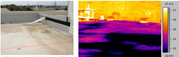
Pulled away wall flashing on Winn Dixie roof
