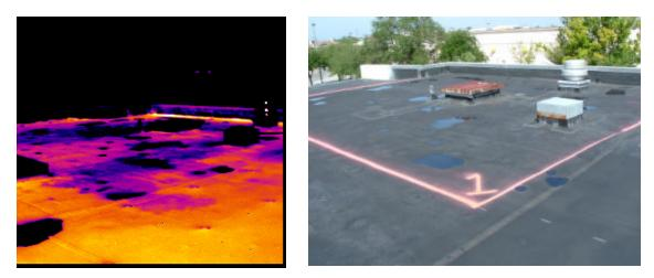
"Cold" thermal anomalies imaged on EPDM roof (at left) during daytime scan. Black areas in thermogram are caused by standing water
